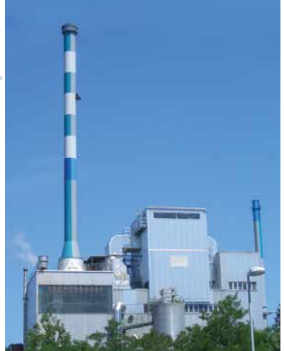
© Luhr Filter. Biomass Combustion plant. Reproduced with kind permission.
