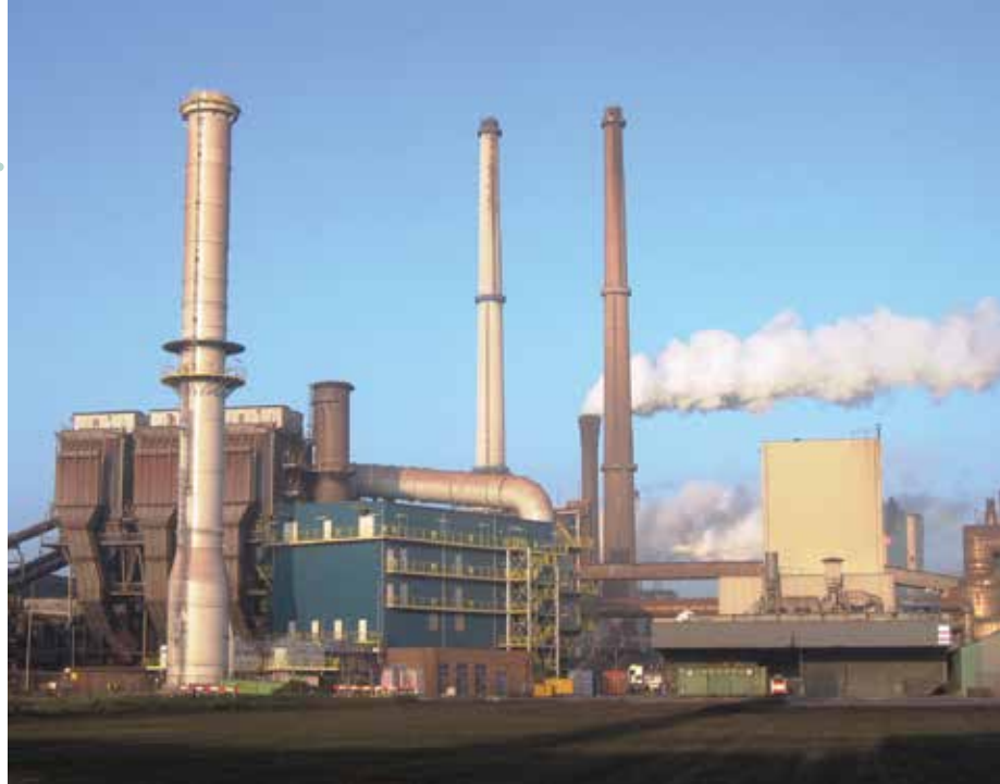
© Luhr Filter. Integrated Steel plant. Reproduced with kind permission.
