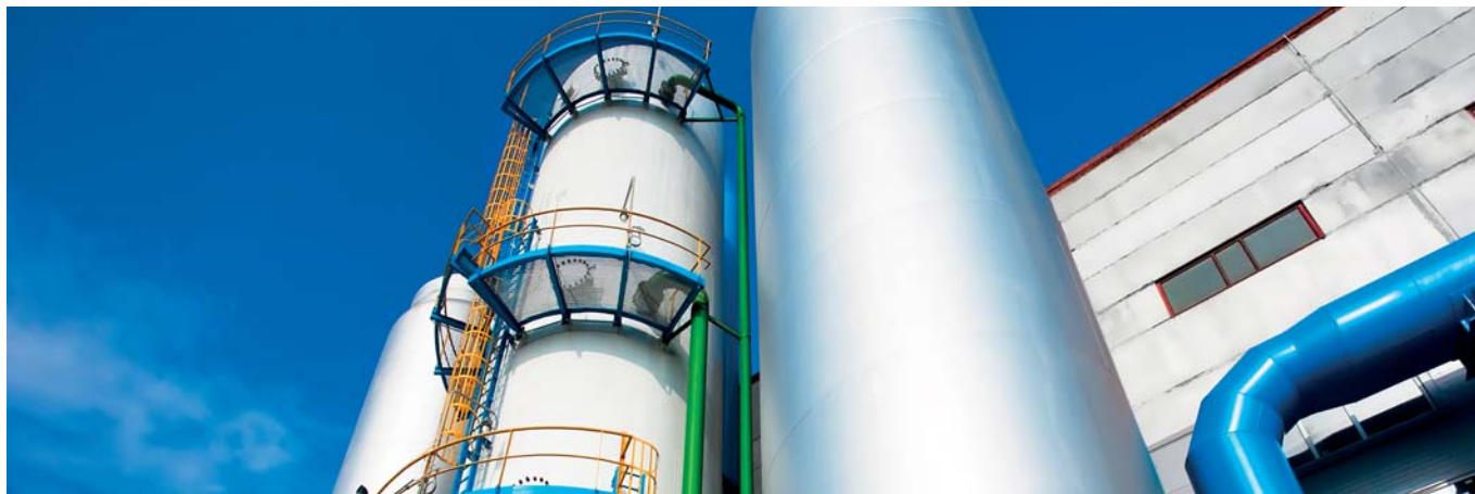
Air Separation Plant
