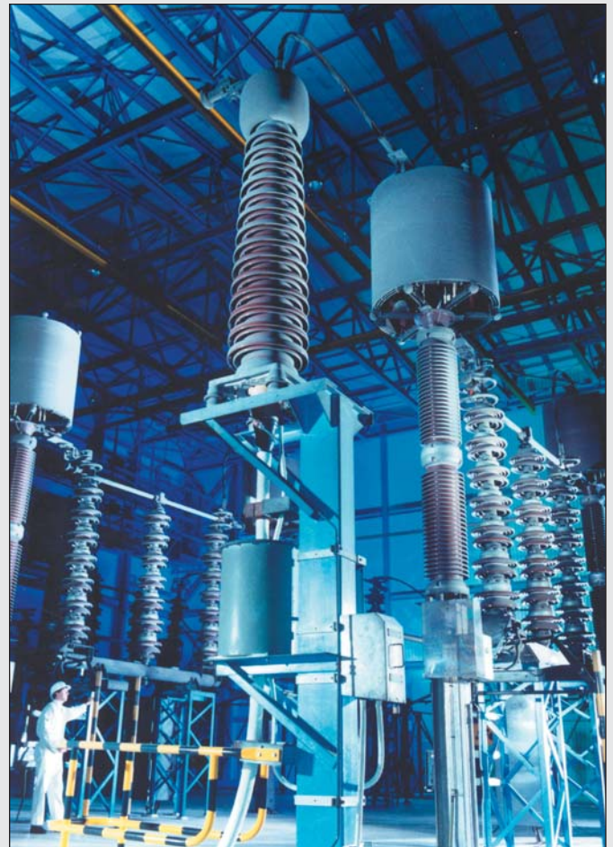
Power station (Peterhead CS)
